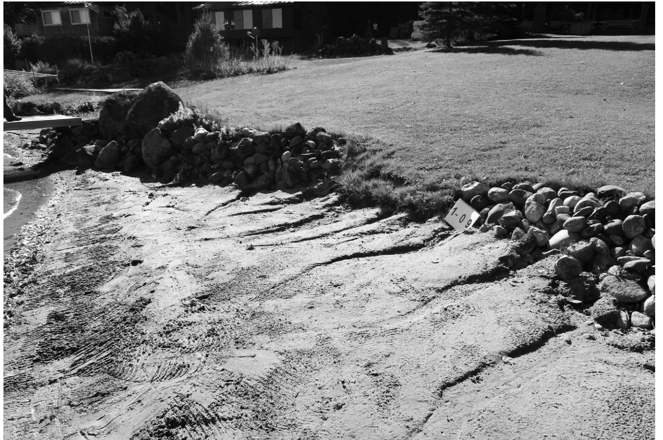
This erosion on McGrath Pond-Salmon Lake is from water flowing across a sloping lawn with no other vegetation to slow the runoff. Grass does not absorb runoff well and is less effective at holding dirt in place.
