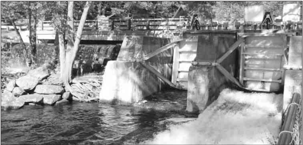
3” flow over the stone spillway
